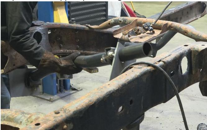
With the remaining two backing plates, push them onto the crossmember ends on the outside of the frame rails, and tac weld them into place.
