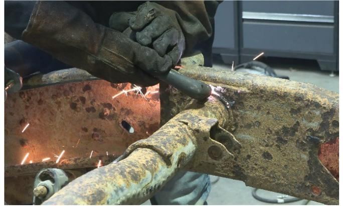
You may find it easier to remove the section by cutting the part in half.
