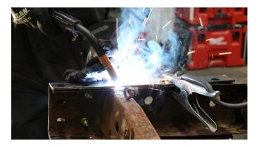
Make sure to weld completely around all edges to prevent future rust and corrosion to the frame rail.
