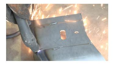
Paint the work area with a weldable primer to help prevent against rust formation.
