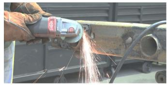
Once the rust and been grinded away, spray the area with a weldable primer to prepare the frame rail for installation.
